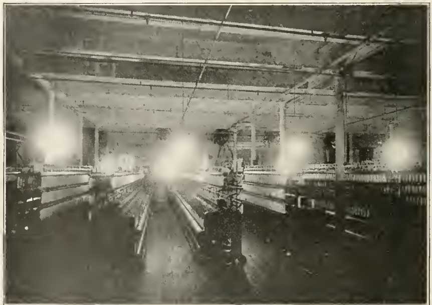
Spinning mill having drop cords with bare lamps. The lighting is very poor and causes eye strain.
